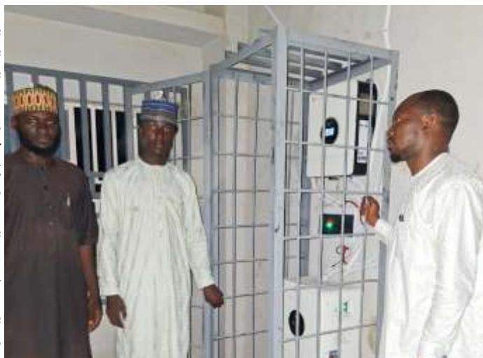
Dean Student Affairs, Prof. Mukhtar Ridwan Bunza inspecting the newly installed solar
